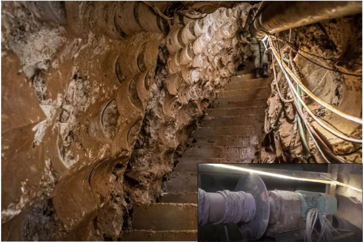
Figure 4: Drilling machine used by Hezbollah in cross-border tunnel that was exposed by the IDF.
