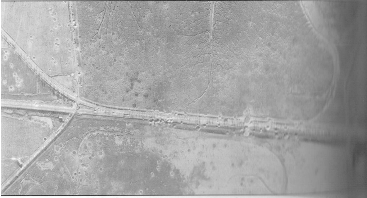
Walcheren causeway with extensive artillery fire damage Source Mark Zuehlke
